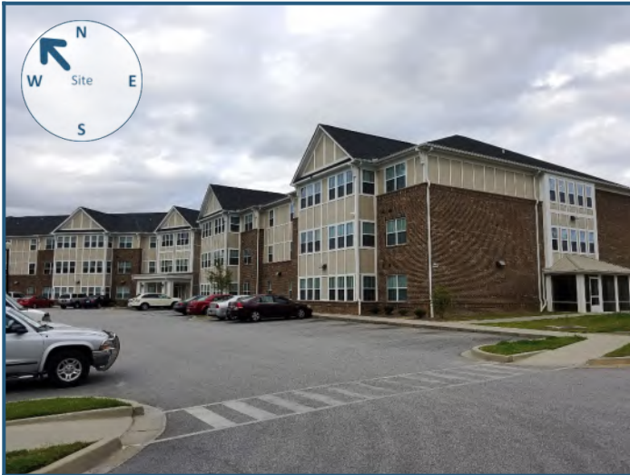
Northwest view from site
